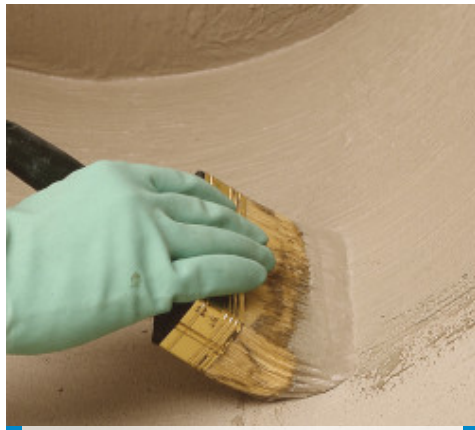
Waterproofing of details by brush
