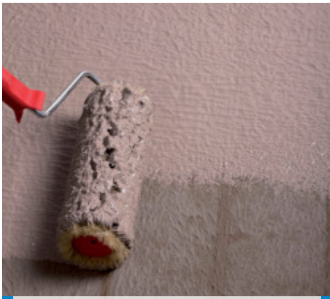
Waterproofing of details by roller
